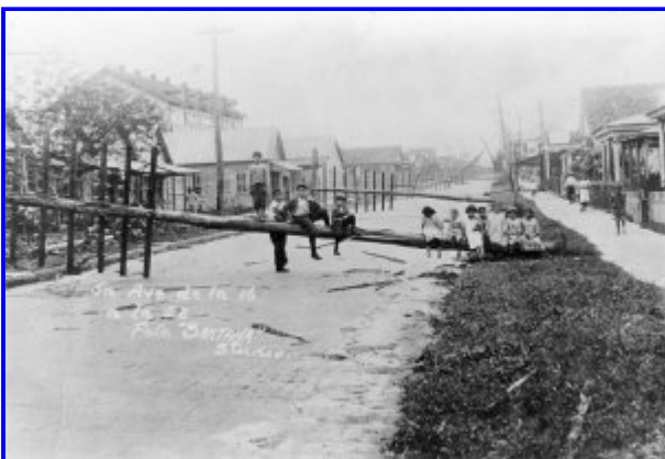
Fallen telegraph poles, Ybor City, Tampa, October 1921 (University of South Florida collections)
