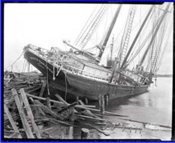
Hurricane damage, Tampa dock, Florida, October 1921 (Photograph: Burgert Brothers collection, Tampa)
